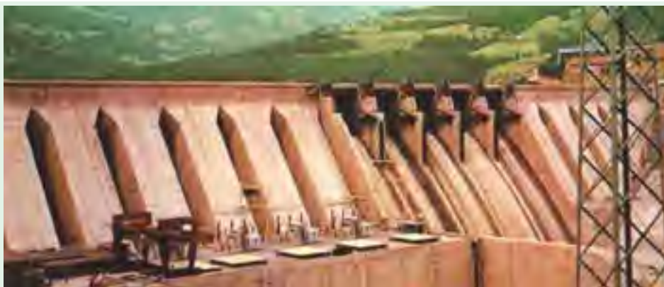
An overview of a hydroelectric plant
