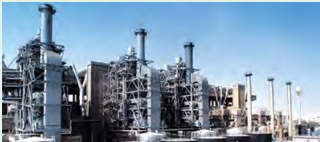
An overview of a thermal power plant
