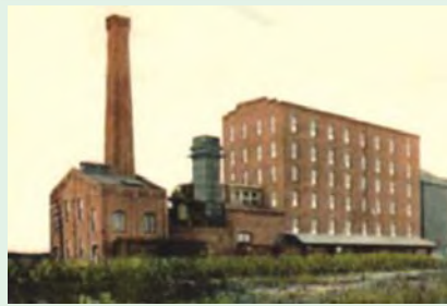
A factory needs electric power for lighting and running motors
